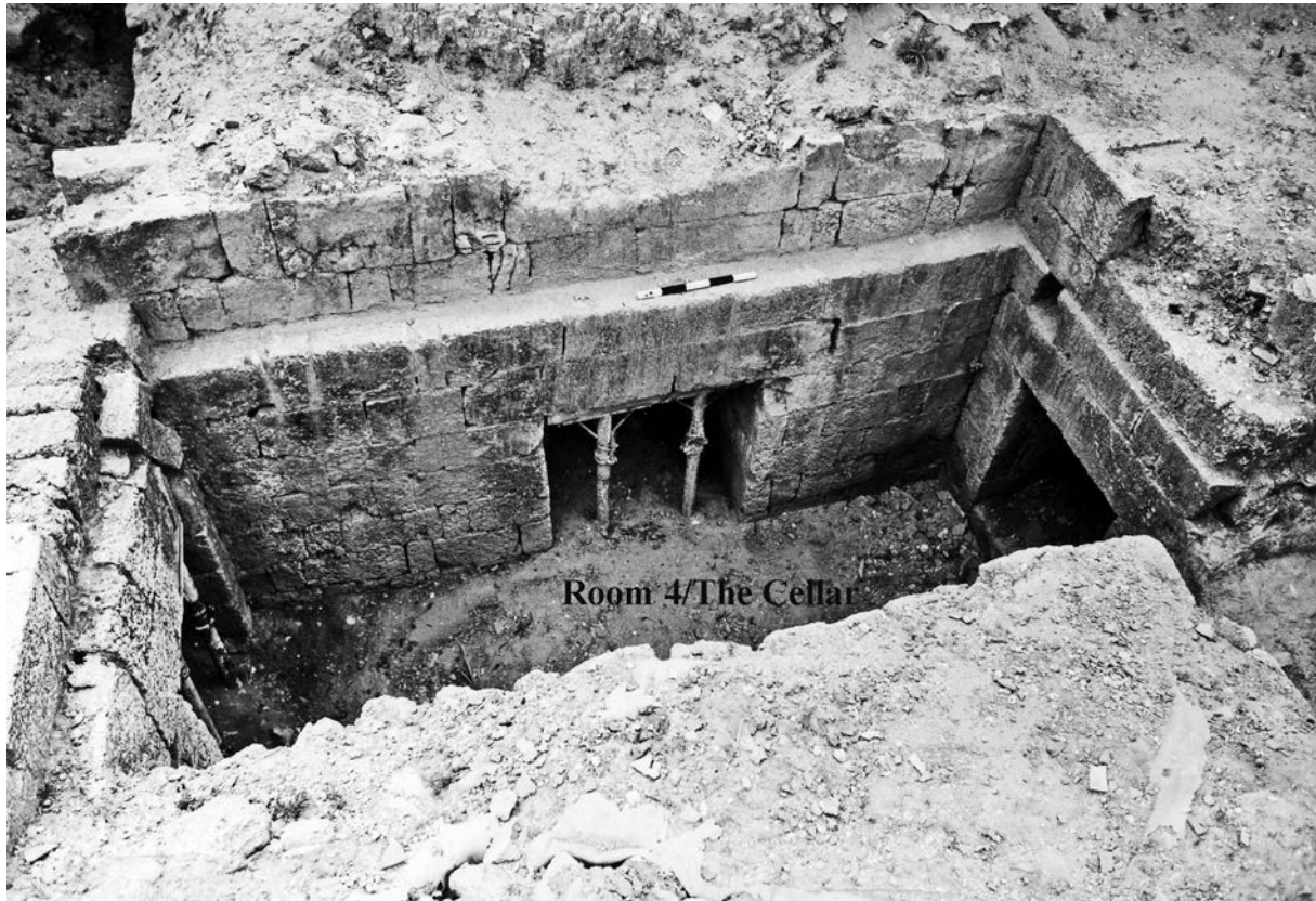
Figure 3.11. Room 4 (the cellar/entrance to catacomb complex). Kaplan Archive.
